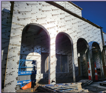
Main entrance south side facing church
