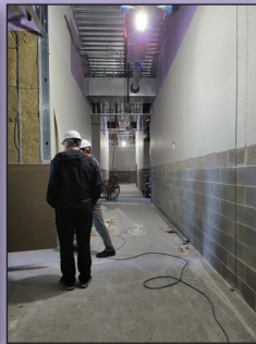
First floor hallway
