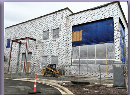
West side view
